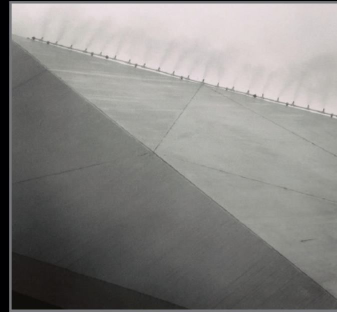
ART MEETS TECH: Artist Fujiko Nakaya and physicist Thomas Mee created artificial fog by spraying pure water through narrow nozzles installed on the Pepsi Pavilion's roof [above left]. The system tracked wind speed and direction [above right] to ensure the fog was distributed over the building's surface. On the pavilion's terrace, autonomous white “floats” built by sculptor Robert Breer [kneeling, below left] roamed about, emitting soft sounds [below right].
